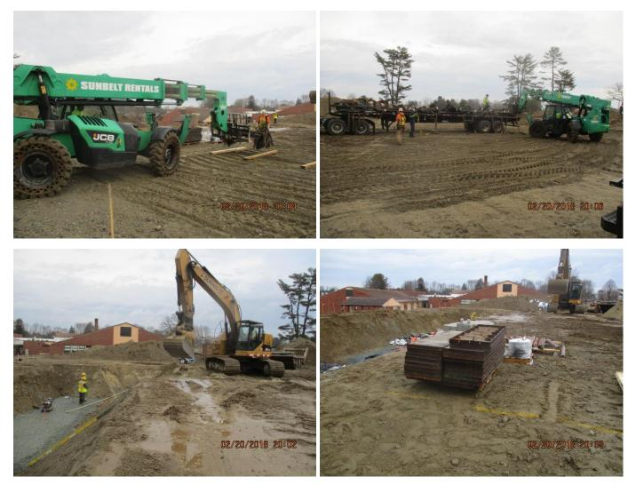
Trucks will be delivering steel and rebar this week. Footings will be poured. Forms and rebar for the foundations will start this week as well. Pictures show rebar and forms delivery and excavation for the foundation start.
