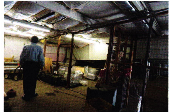
DPW Mezzanine Loft – note vapor barrier failures
