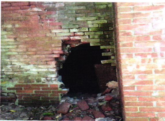
Masonry damage on Northwest wall
