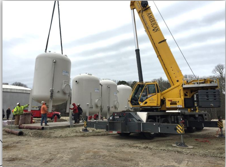
Example of Full size GAC contactors being installed
