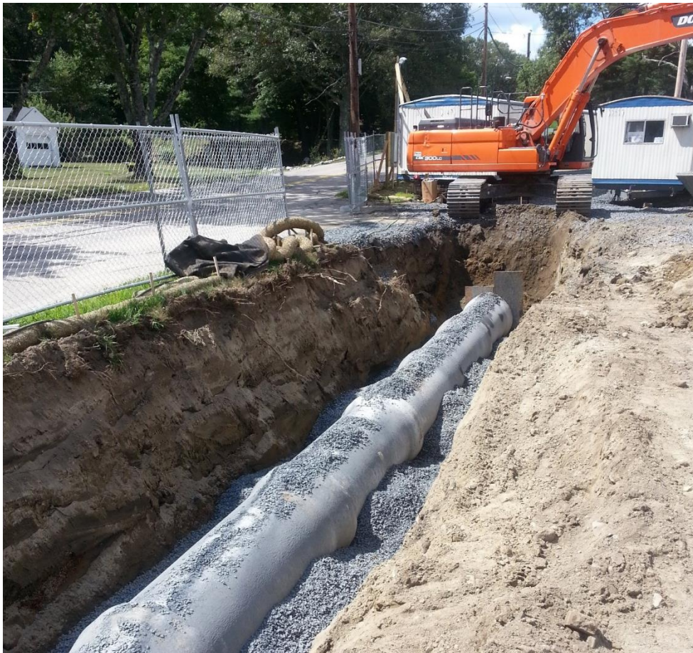
New 30" Drainline installation 8-10-15
