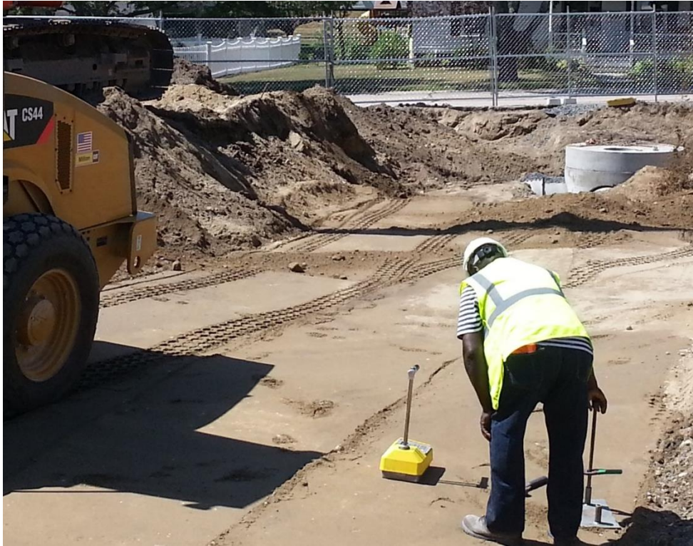
Compaction Tests over Backfilled Drainline under Parking Lot 8-19-15
