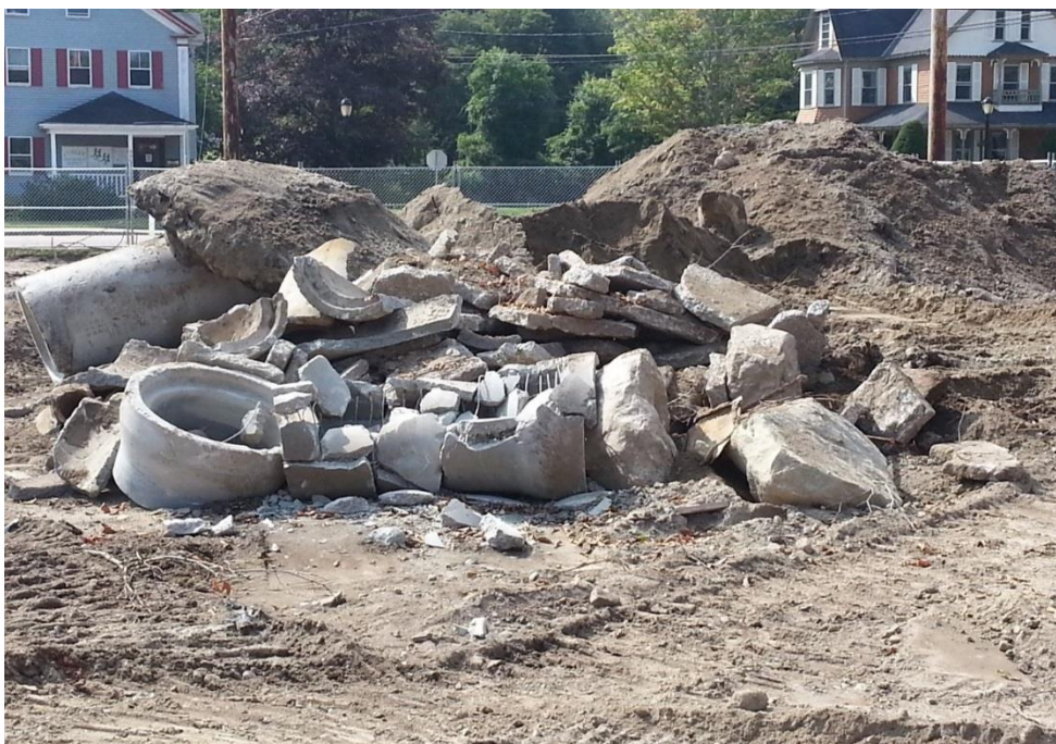
Demolished 24" RCP Culvert 8-18-15
