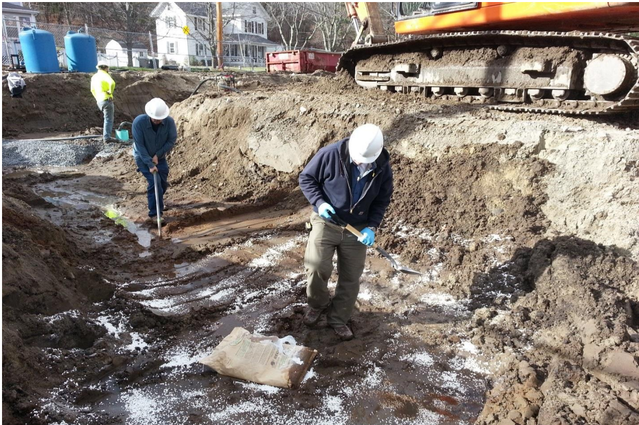
CREWS APPLYING OXIDIZER AT PETROLEUM MITIGATED AREA 12-3-15
