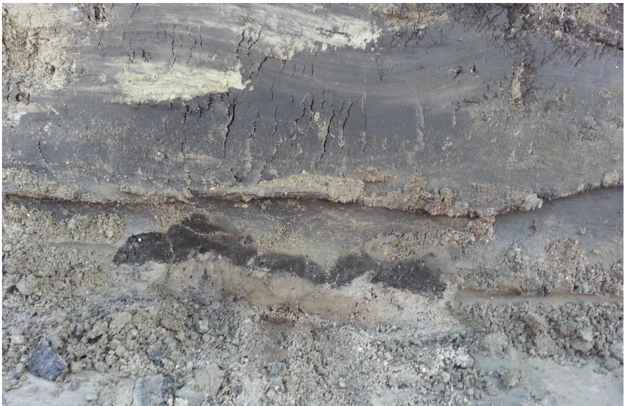
2.5 to 3 FOOT LAYER OF ORGANICS IN GARAGE FOOTING LINE 12-23-15
