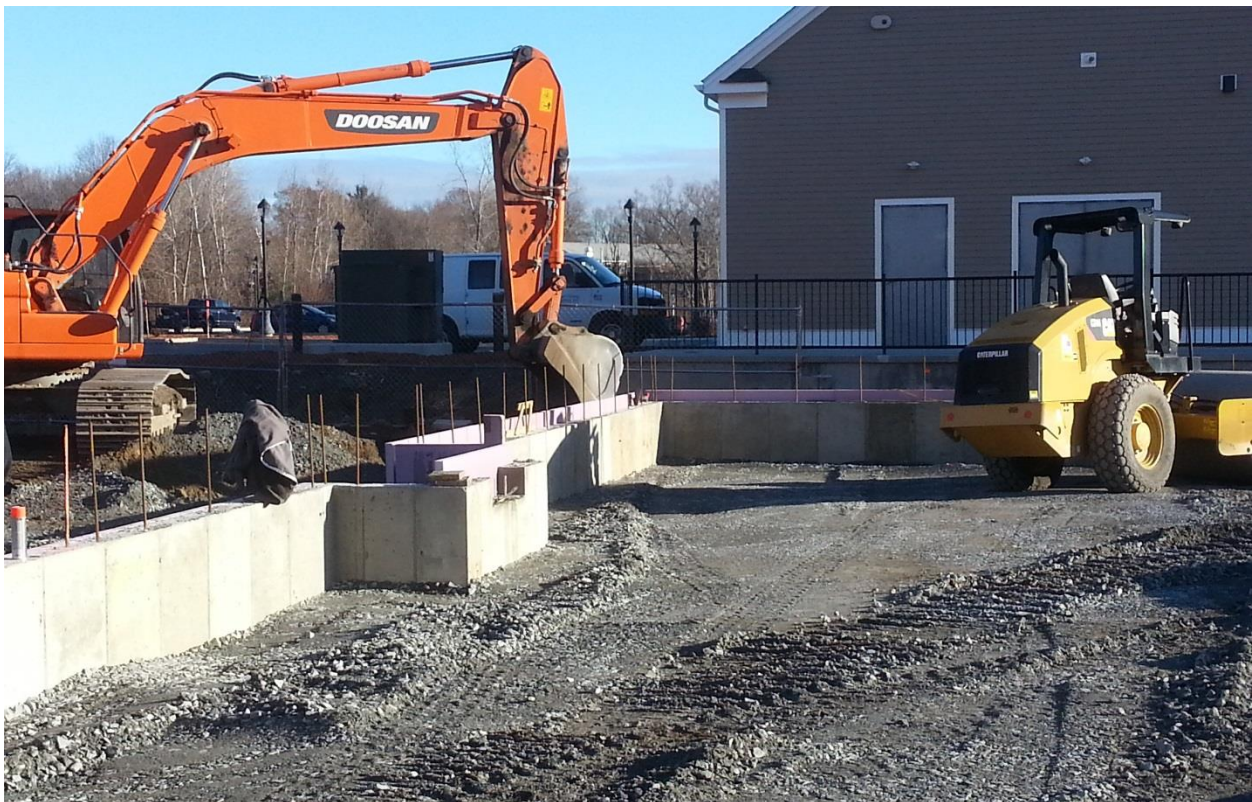
FOUNDATION BACKFILLING 12-16-15
