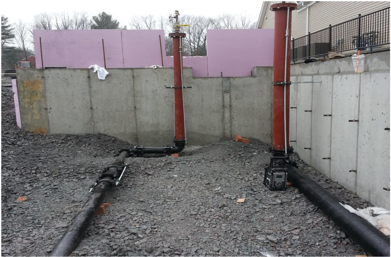
FIRE PROTECTION & WATER SERVICE RISERS 12-21-15
