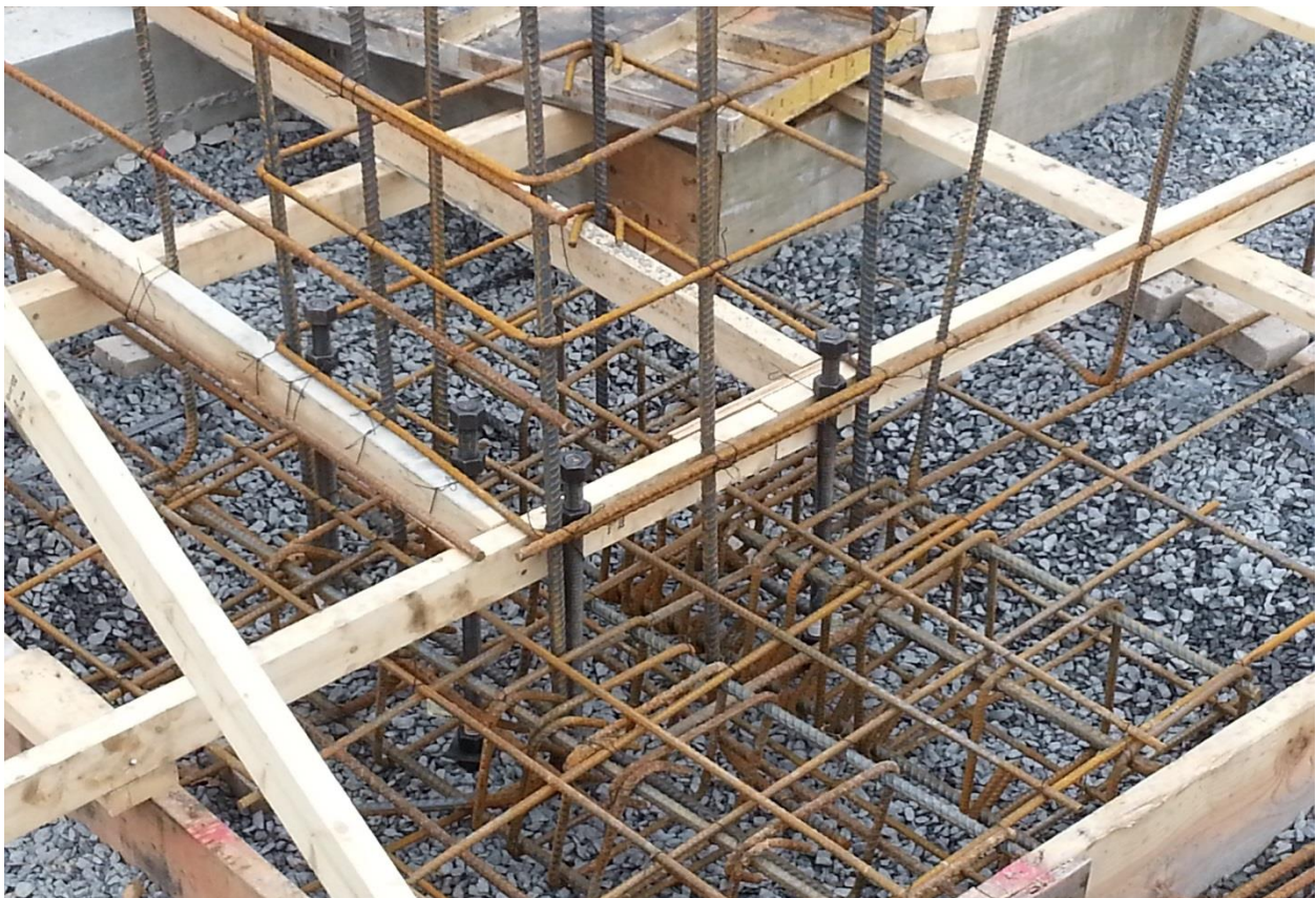
TOWER PIER FOOTING WITH SHEAR WALL ANCHORS 12-21-15
