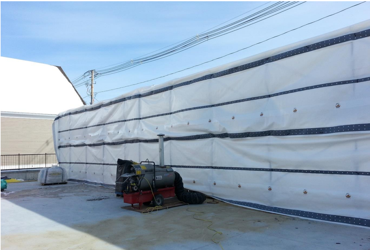
MASON'S TEMPORARY ENCLOSURE 2-12-16
