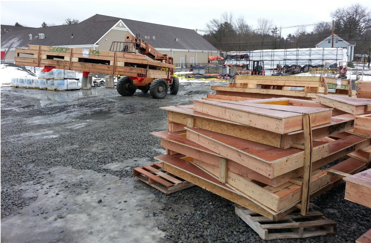
PRE-FABRICATED WALL PANEL DELIVERY 2-16-16
