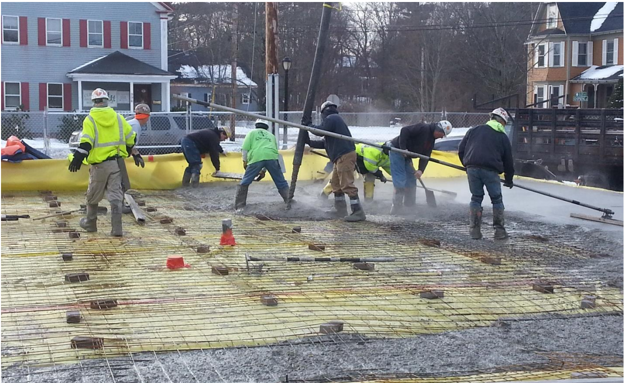
PLACING CONCRETE SLAB 1-26-16
