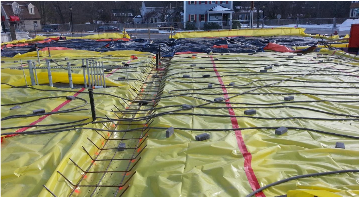
HAUNCH REINFORCING, HEATING TUBES 1-20-16
