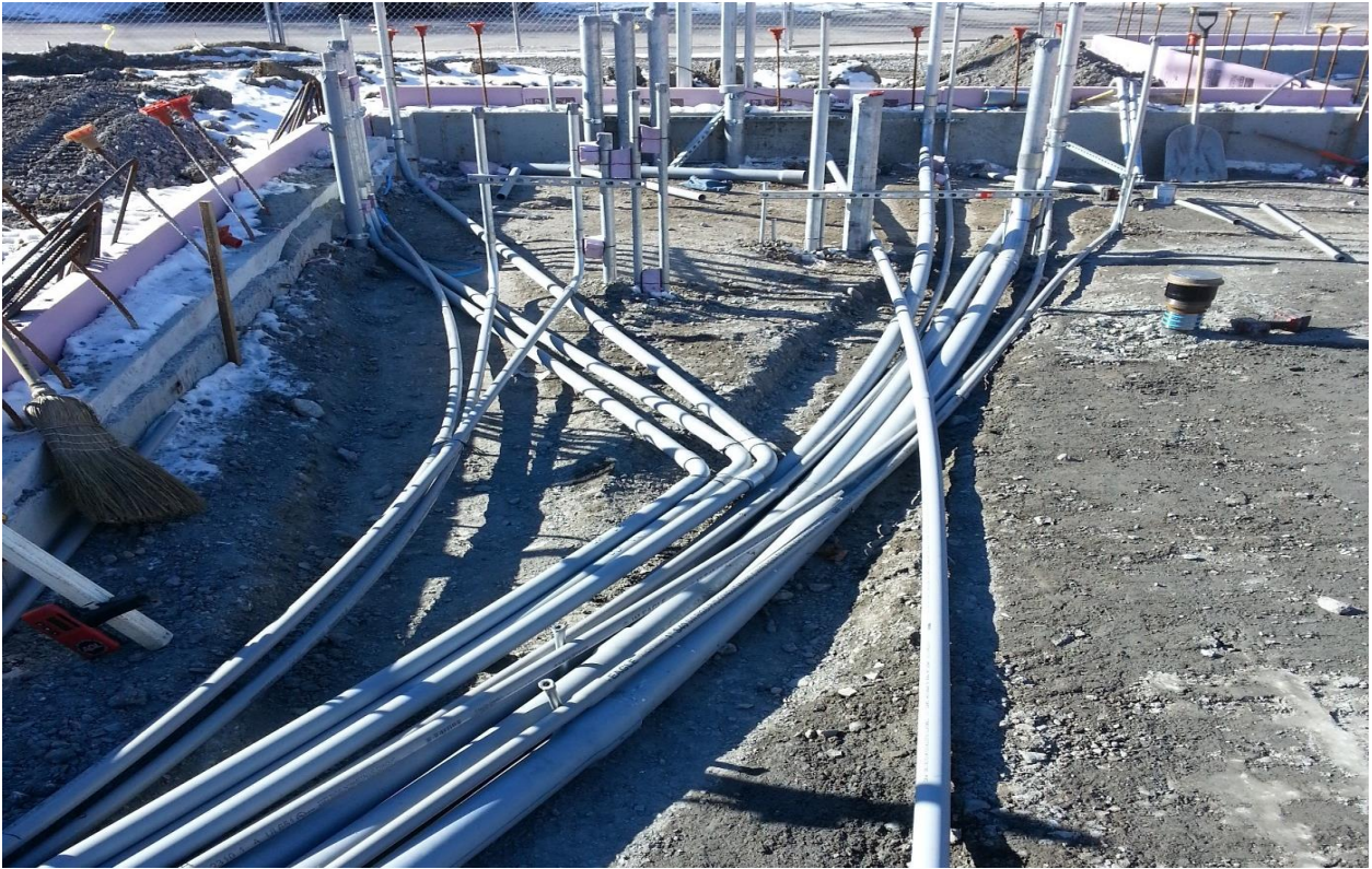
UNDERGROUND ELECTRICAL UTILITIES 1-20-16
