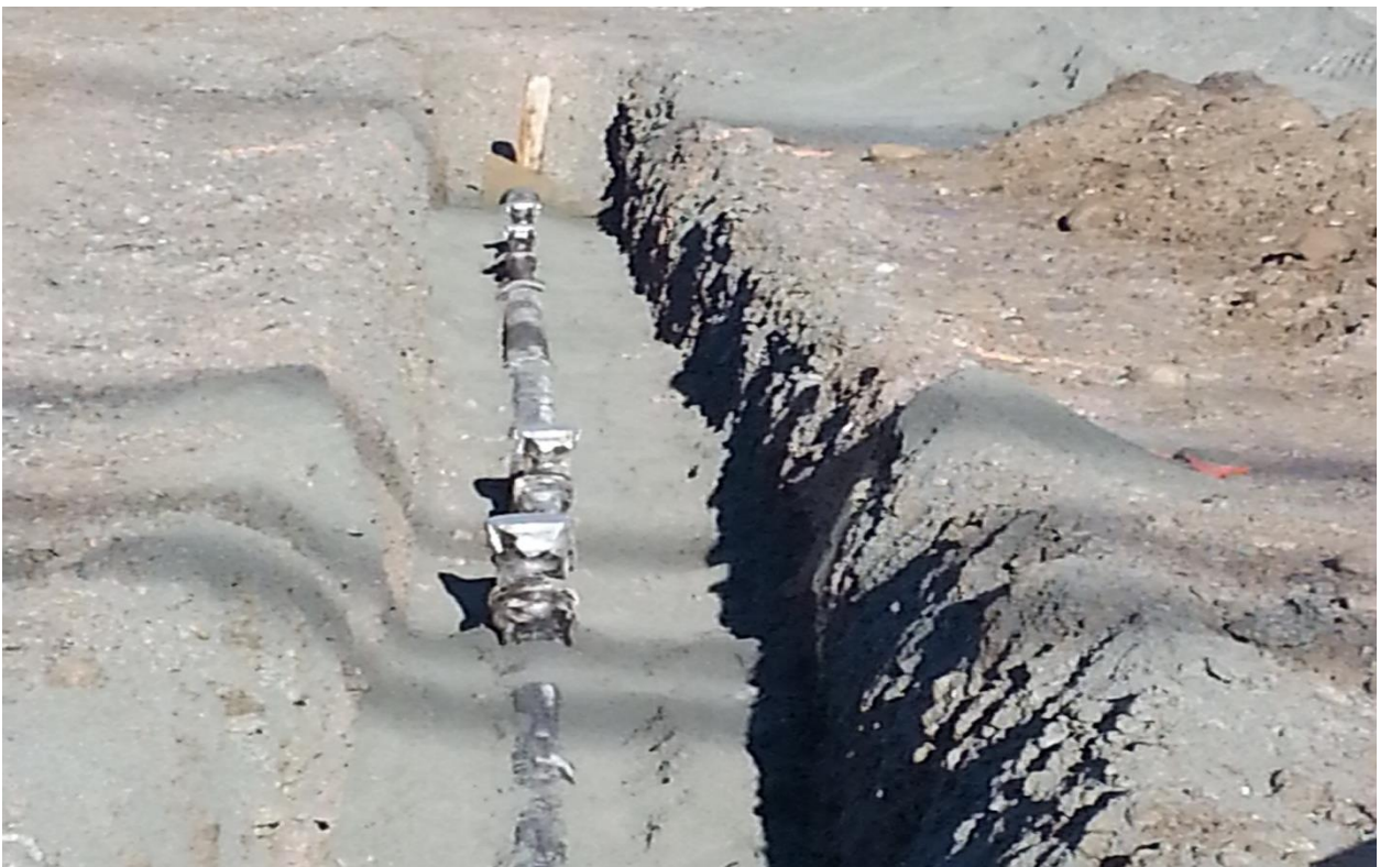
UNDERGROUND PLUMBING LINES 1-4-16
