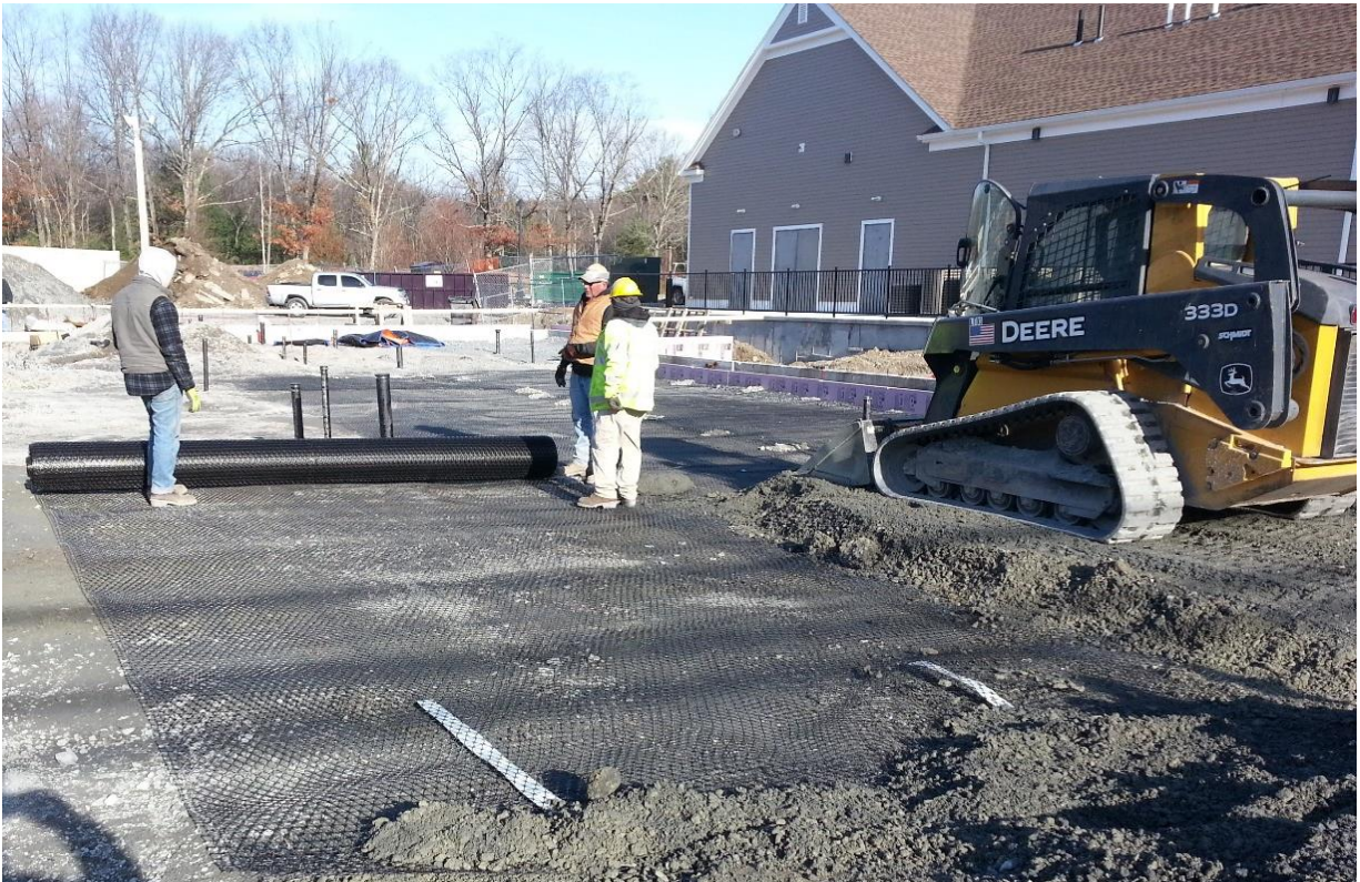
INSTALLING GEO-GRID 1-11-16
