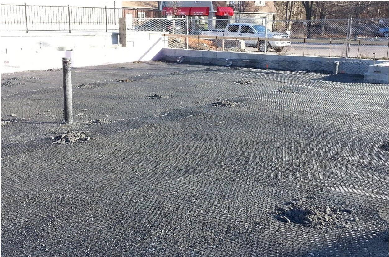
INSTALLING GEO-GRID 1-10-16
