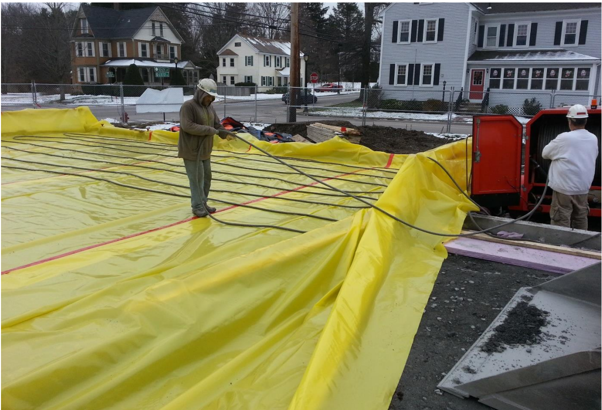
GROUND THAW UNIT & SETTING OUT HEATING TUBES 1-15-16
