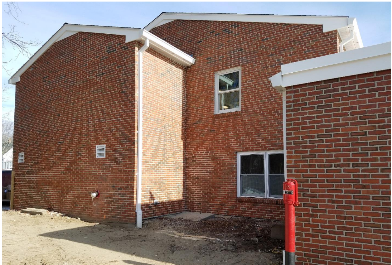
Westside elevation showing new windows, exterior roof trim & PIV in foreground
