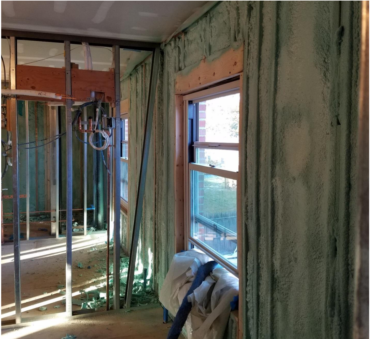
Spray-foam wall insulation
