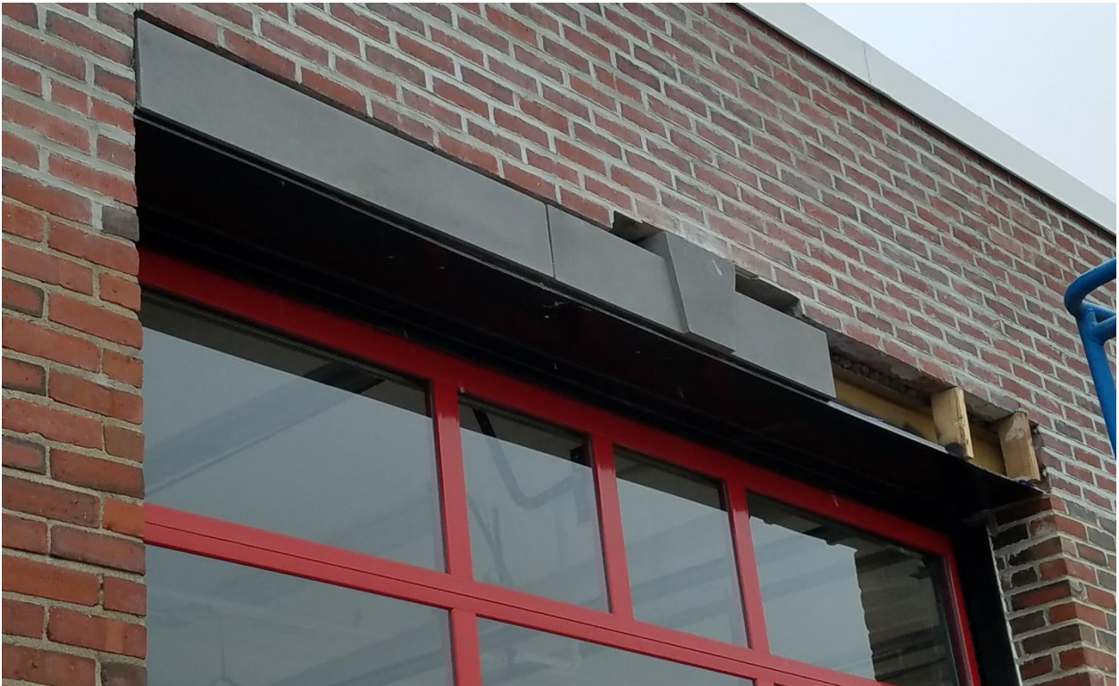
Precast lintels needing structural anchoring
