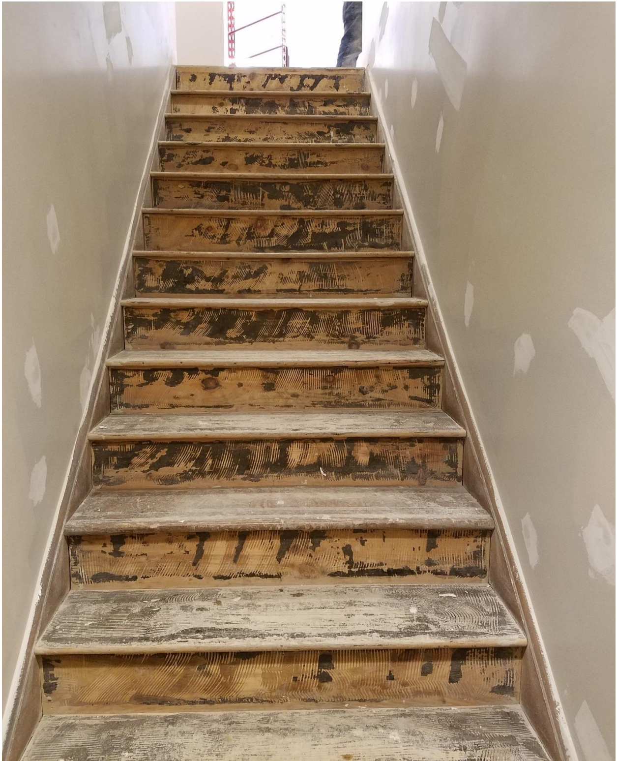
Existing non-compliant stairs to second floor
