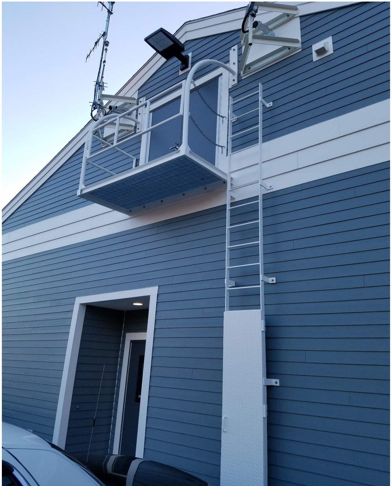
Attic access platform & ladder at MPD
