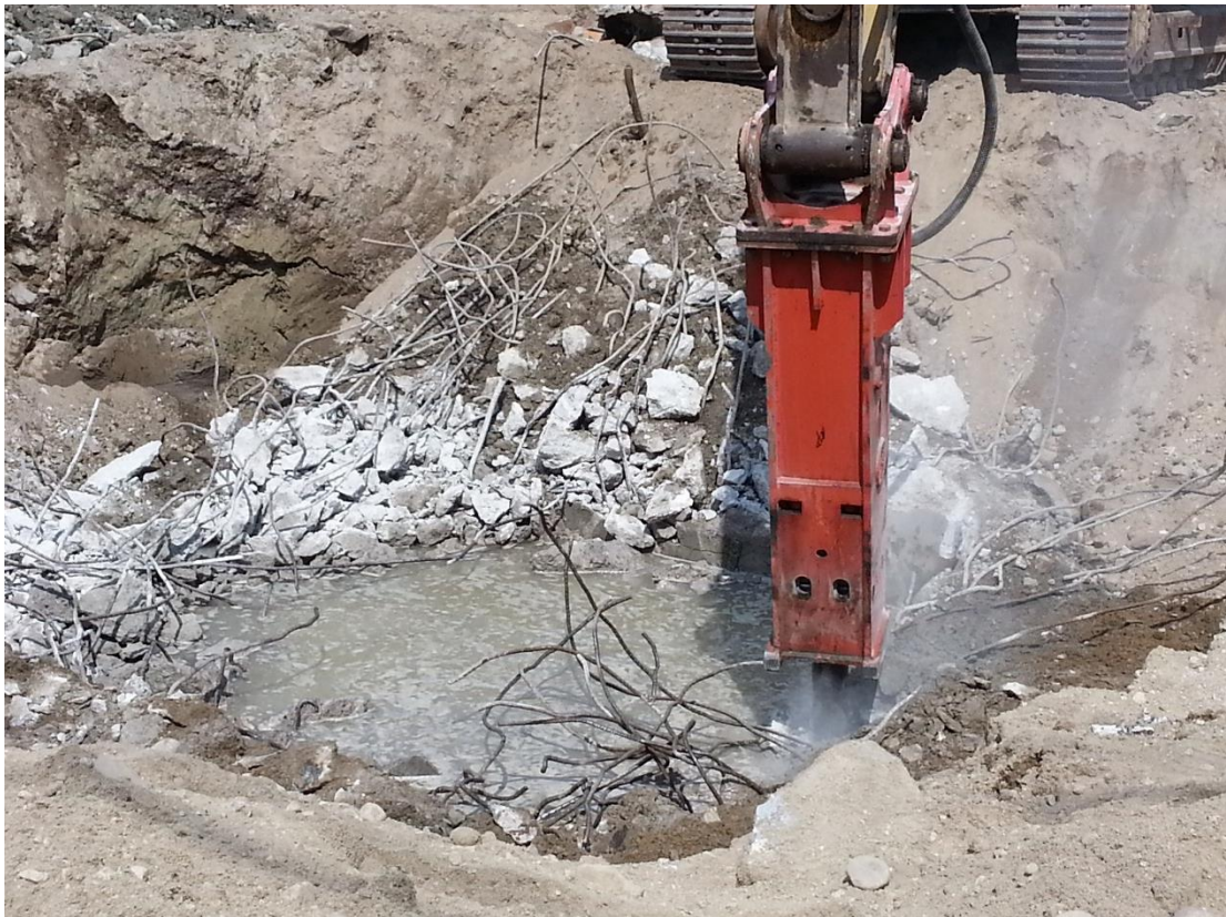
Hoe-ramming existing concrete foundation at old sewer station 7-28-15
