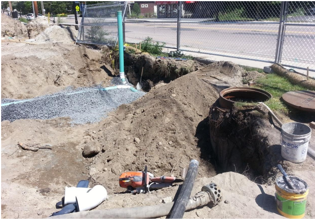
Sewer tie-in to SMH at front yard 7-31-15
