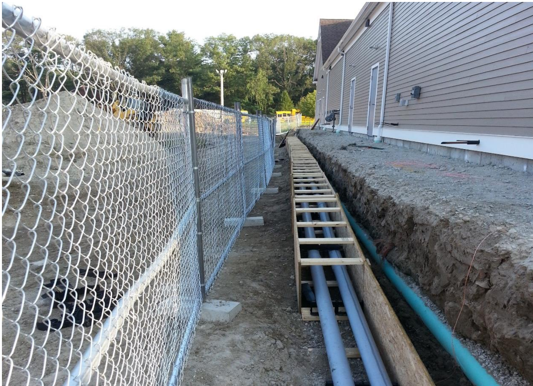
JOPA Property showing electrical ductbank 7-30-15
