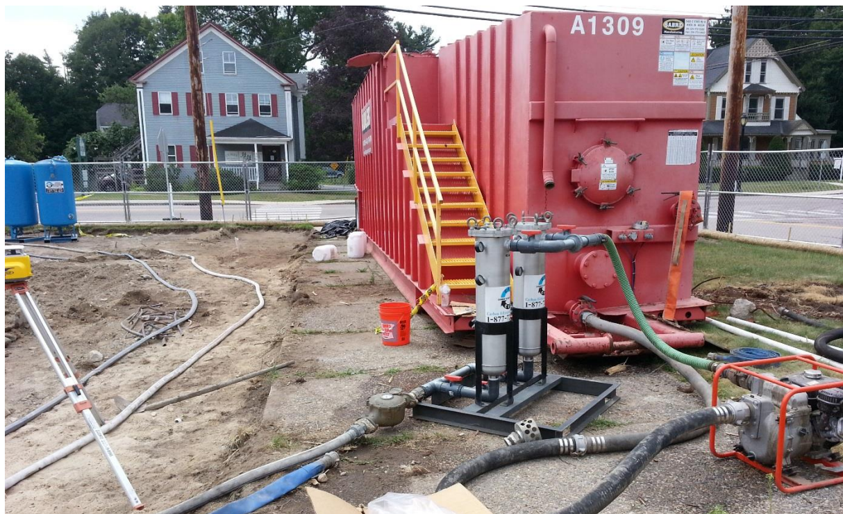
Groundwater filtering system 7-30-15
