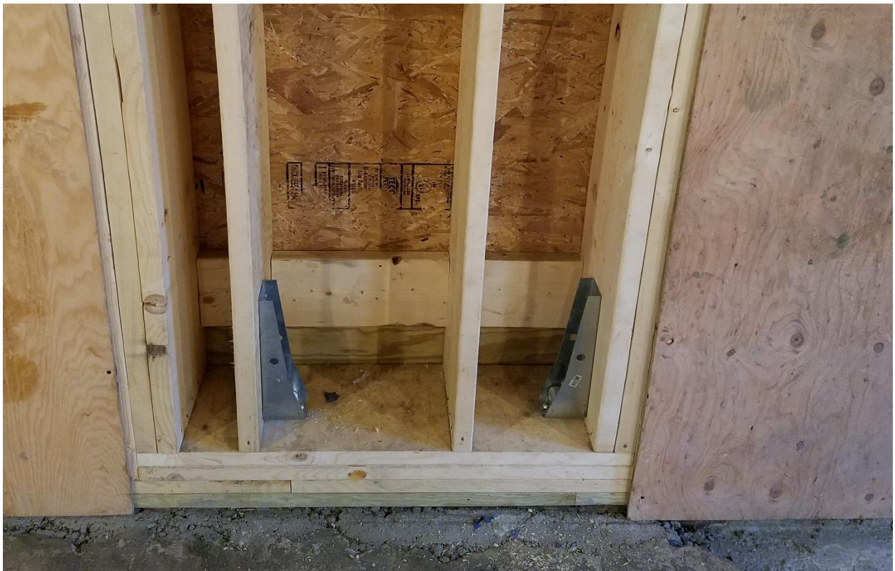
JACK STUD ANCHORS at FRONT WALL 11- 16 -16
