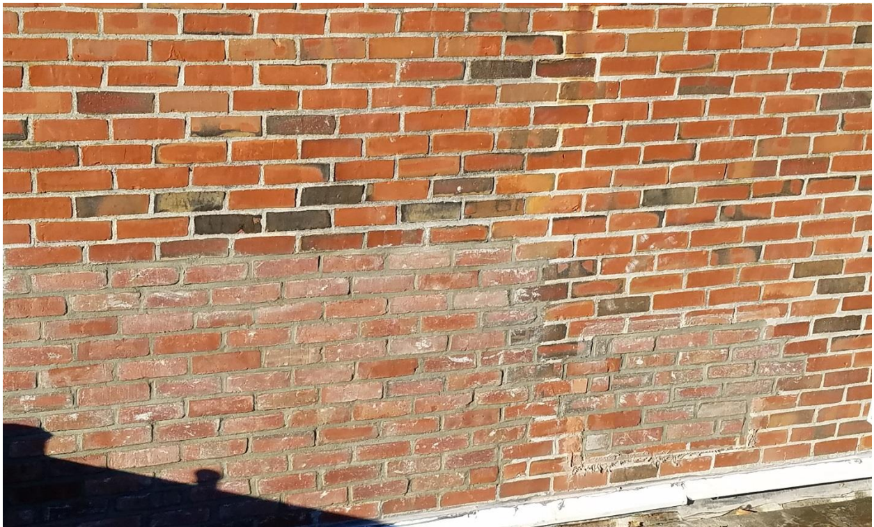
BRICK INFILL AT ABANDONED OPENINGS 11-18 -16
