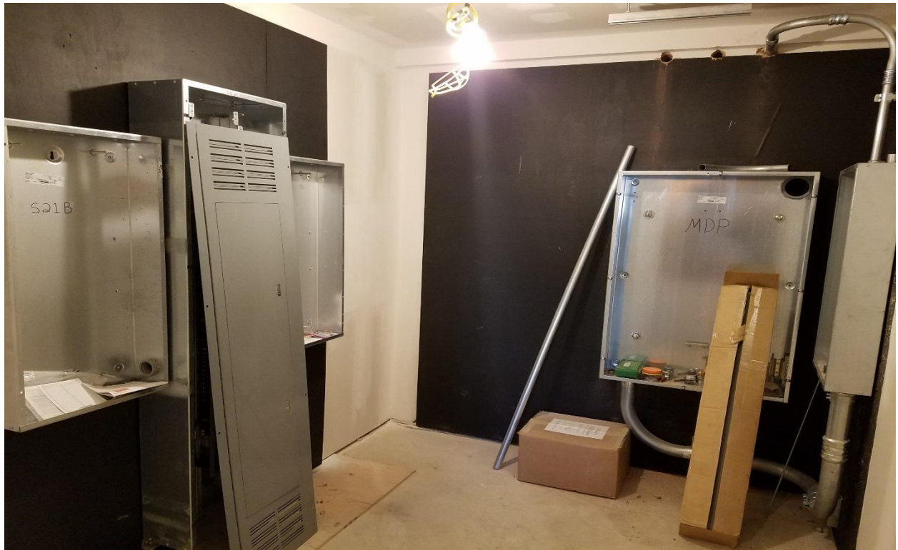
MAIN ELECTRICAL ROOM PANEL TUBS SET 11-21 -16
