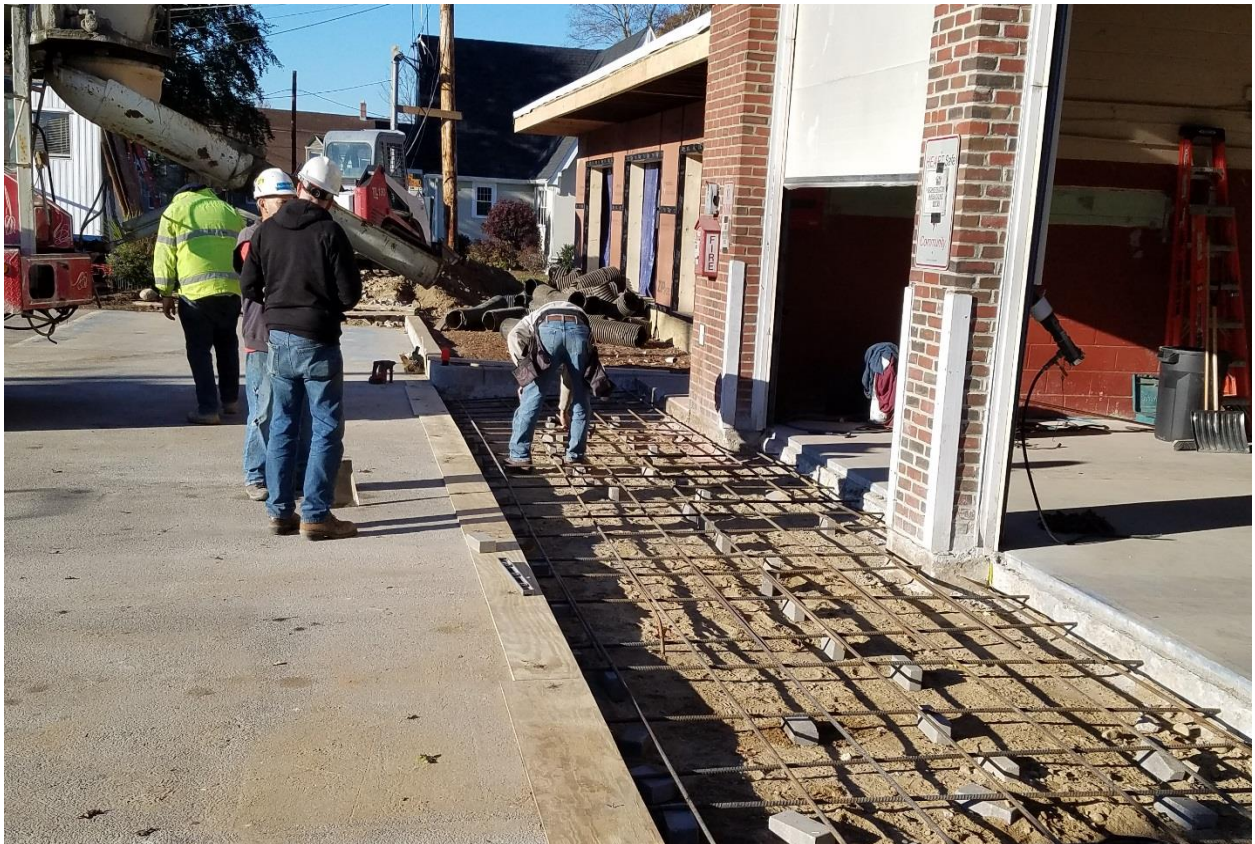
PLACING NEW CONCRETE APRON 11-8-16
