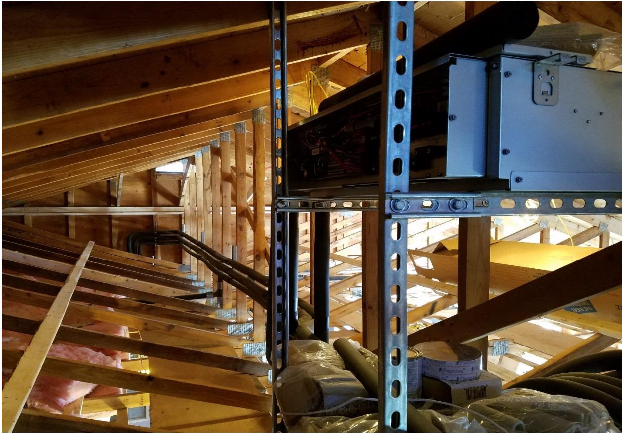
NEW ATTIC TRUSS BRACING & AHU INSTALLATION 11-16 -16
