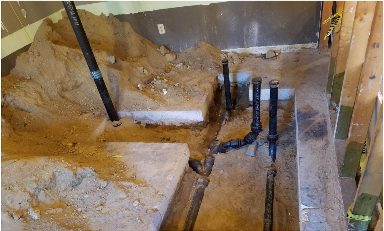
NEW UNDERGROUND PLUMBING 11-2 -16
