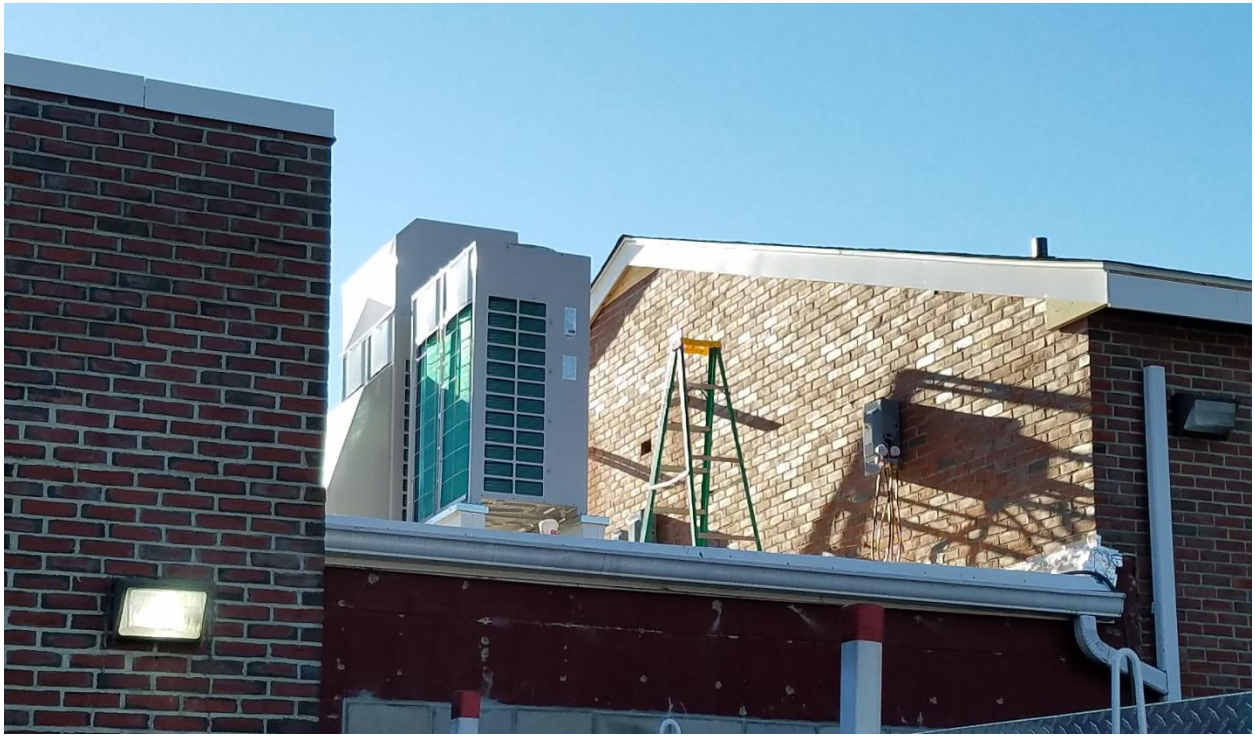
ROOF TOP UNIT SET as viewed from REAR showing NEW ROOF TRIM 11- 30 -16
