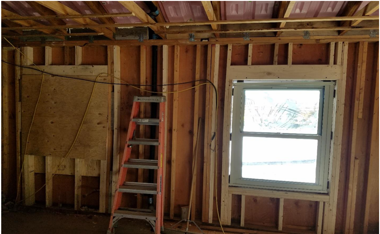
ADDITIONAL STUDS PLACED UNDER EACH TRUSS 11-16 -16
