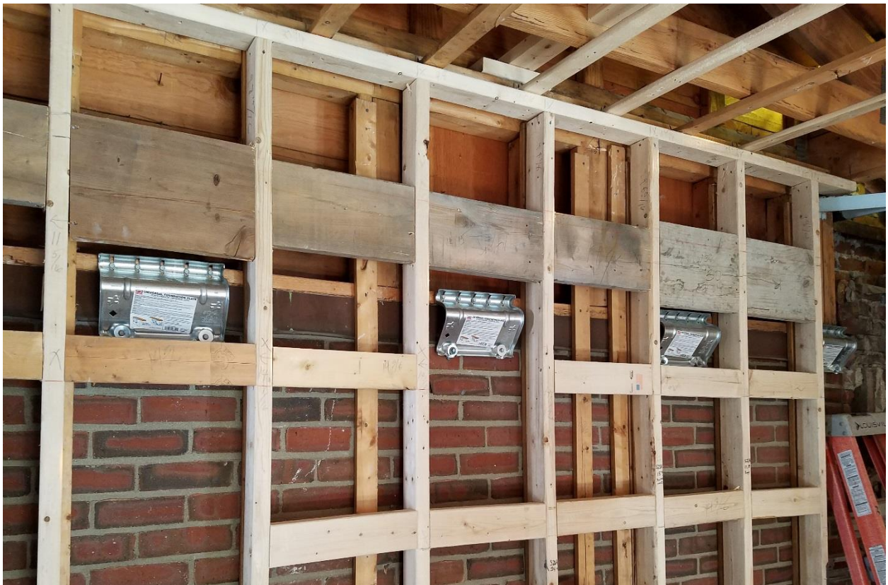
NEW MASONRY WALL-to- WOOD WALL ANCHORS 11-15 -16
