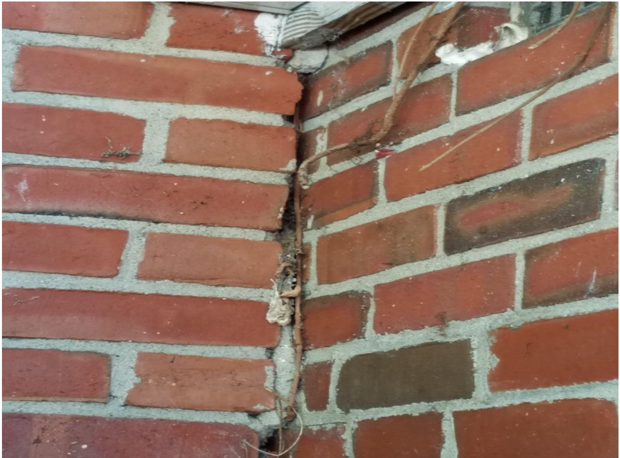
MASONRY NEEDING REWORK AND INSTALLATION OF CONTROL JOINT
