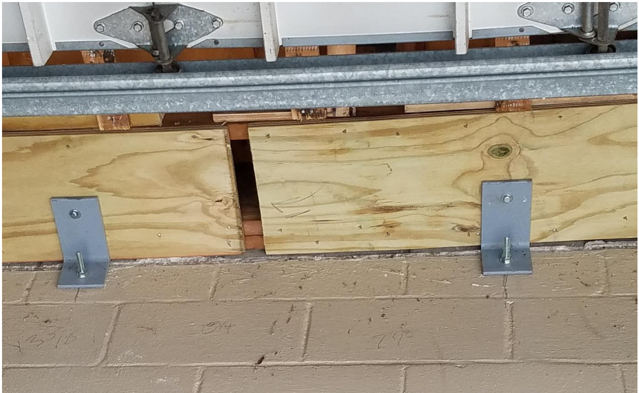
SEISMIC CLIPS INSTALLED AT TOP OF MASONRY WALLS
