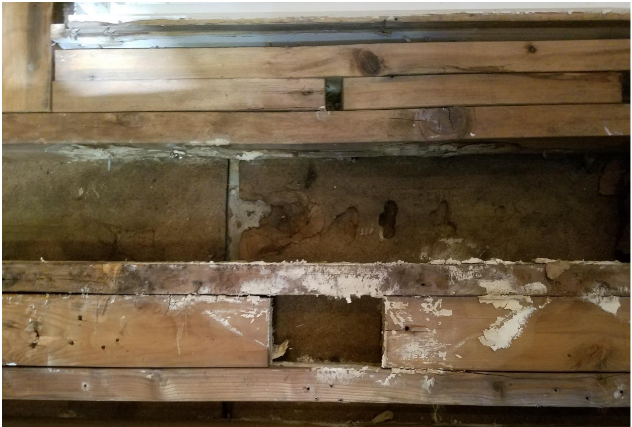
ADDITIONAL AREAS OF ROT & MOLD DAMAGED WOOD FRAMING
