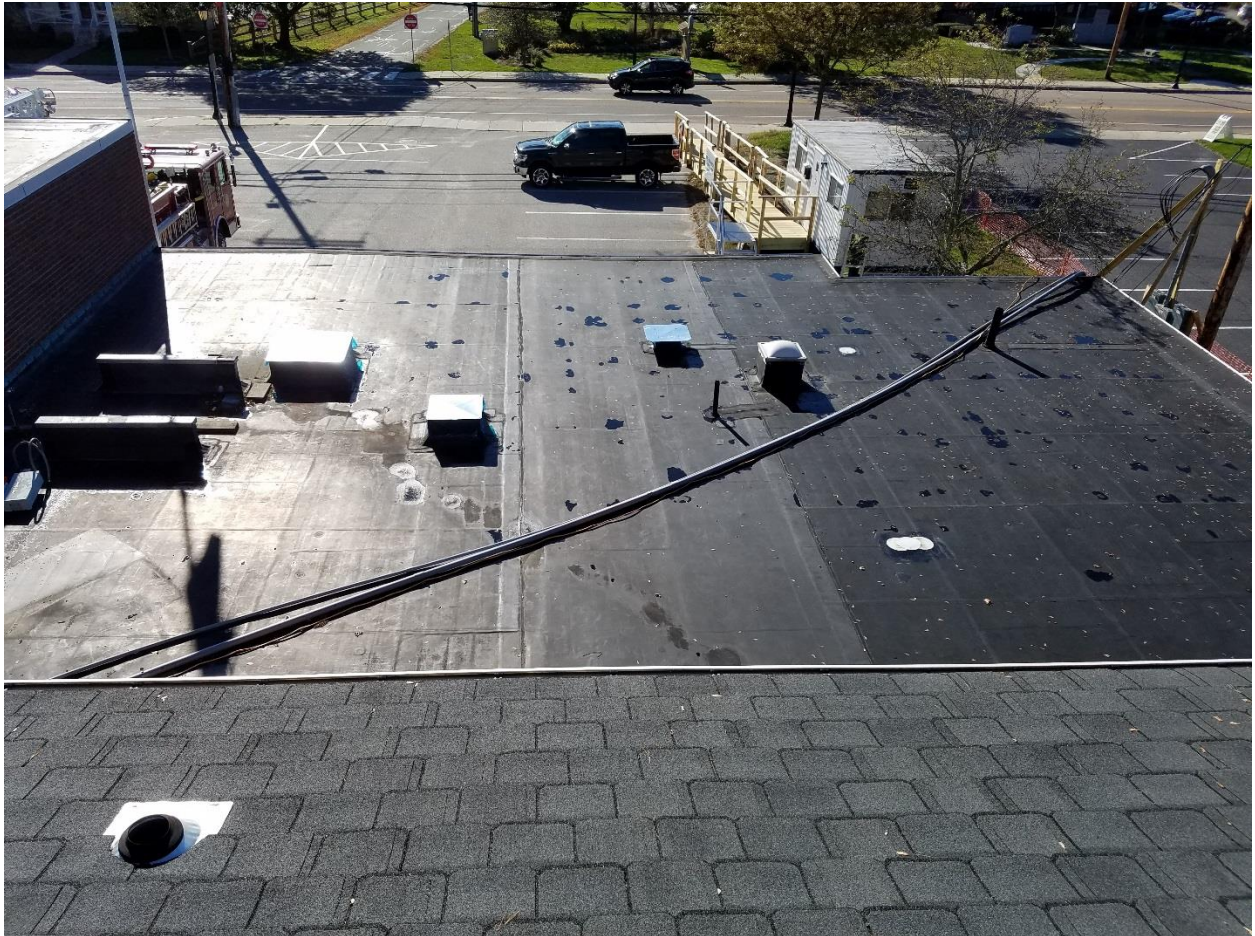
ADMIN MEMBRANE ROOF AREA TO BE REPLACED AS PART OF BASE BID
