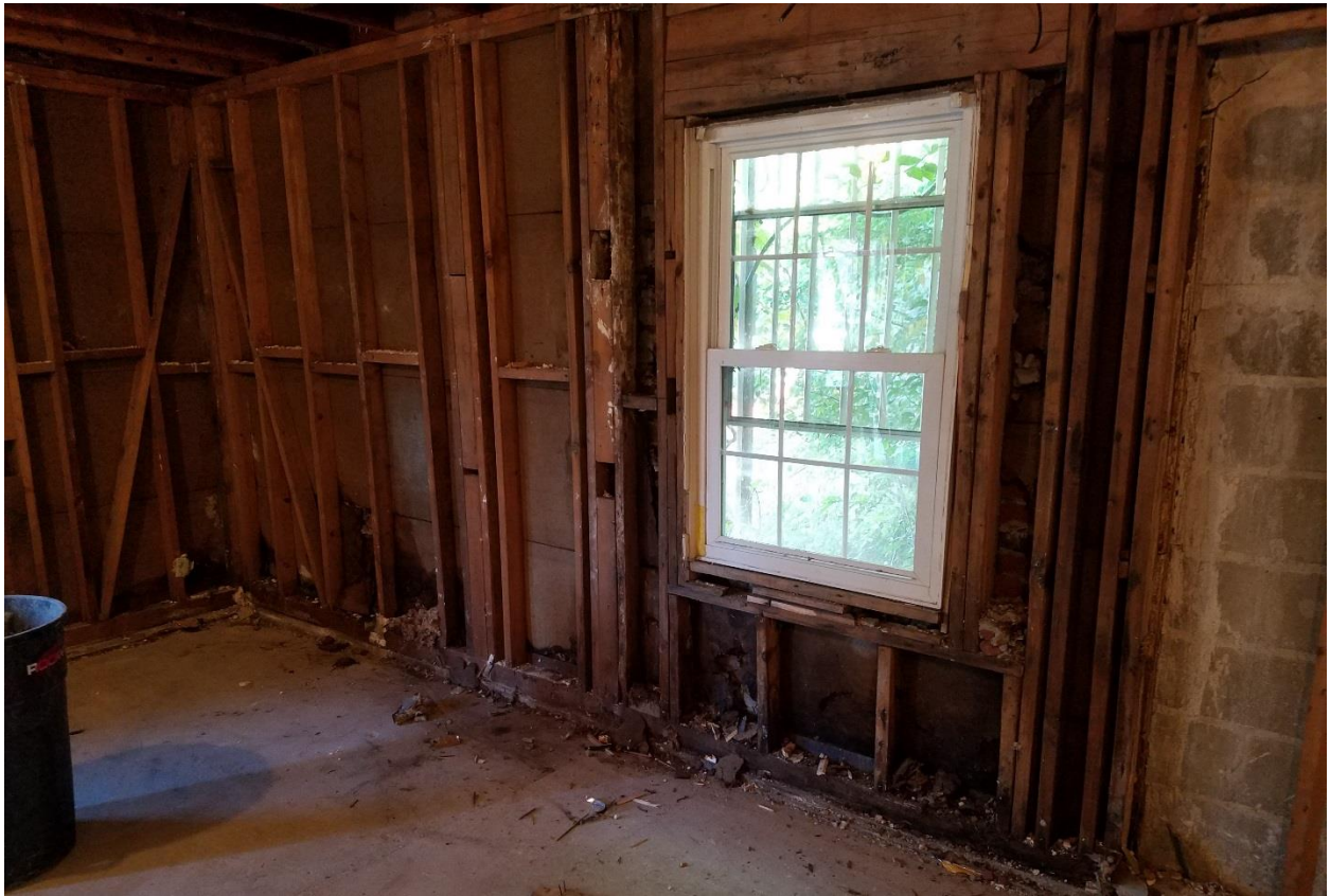
AREAS OF WATER-DAMAGED WOOD FRAMING
