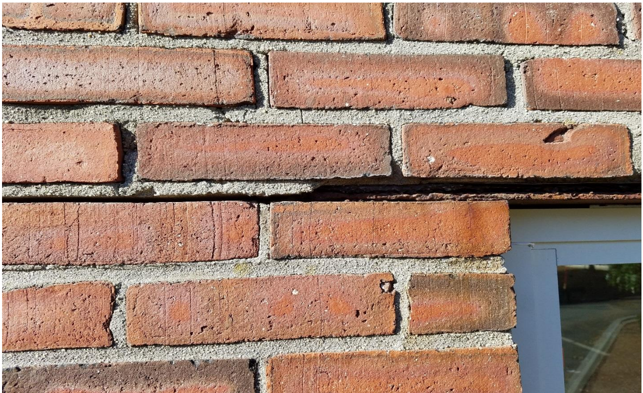
MASONRY JOINTS NEEDING RE-POINTING
