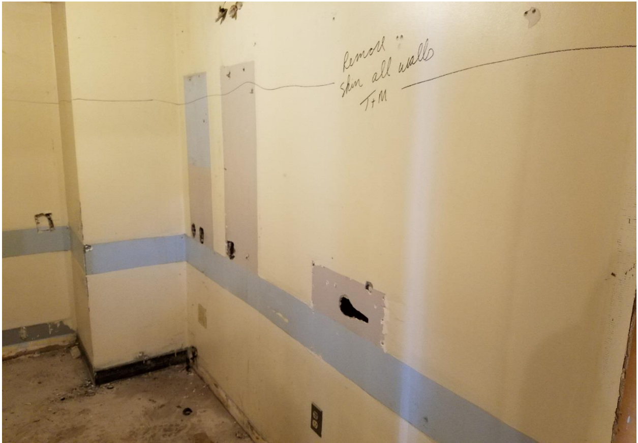
EXISTING SHEETROCK NEEDING DEMOLITION FOR NEW WORK
