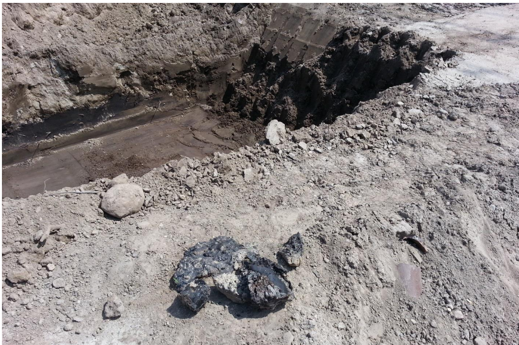
ORGANIC LAYER VISIBLE IN SIDEWALL OF FOOTING EXCAVATION WITH OIL GLOBULE IN FORGROUND 9-1-15
