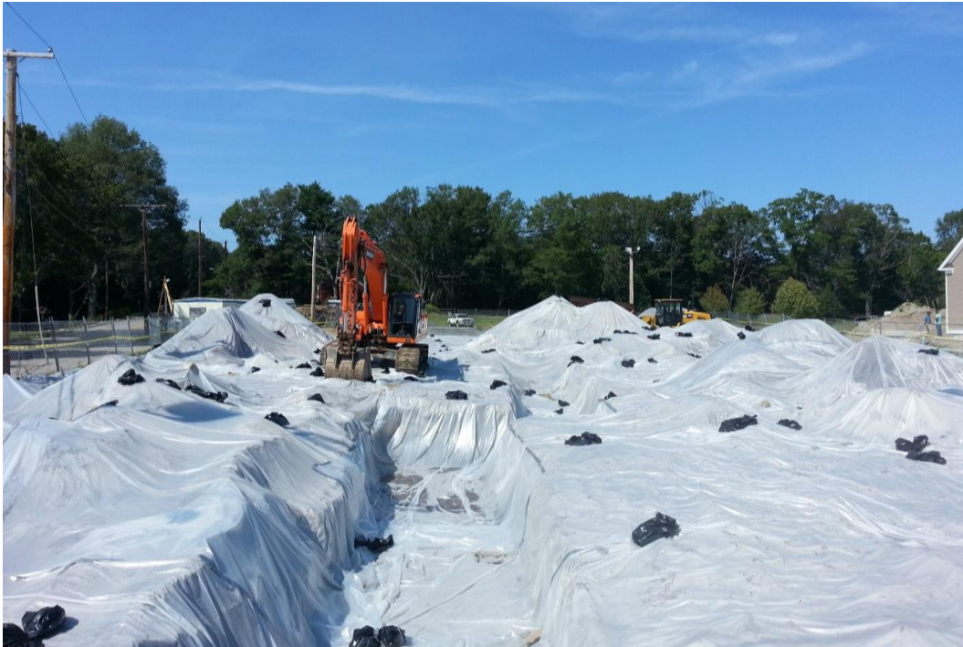
POLYETHYLENE COVERING ALL EXCAVATIONS WITH QUARANTINED EQUIPMENT 9-15-15
