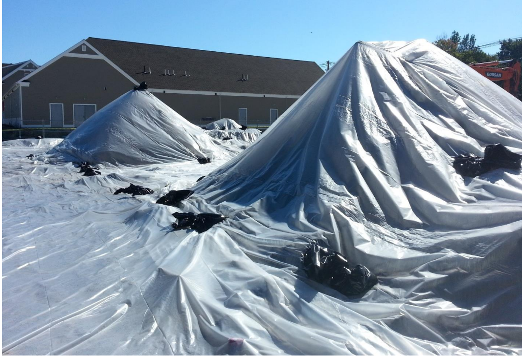
POLYETHYLENE COVERING STOCKPILES 9-15-15
