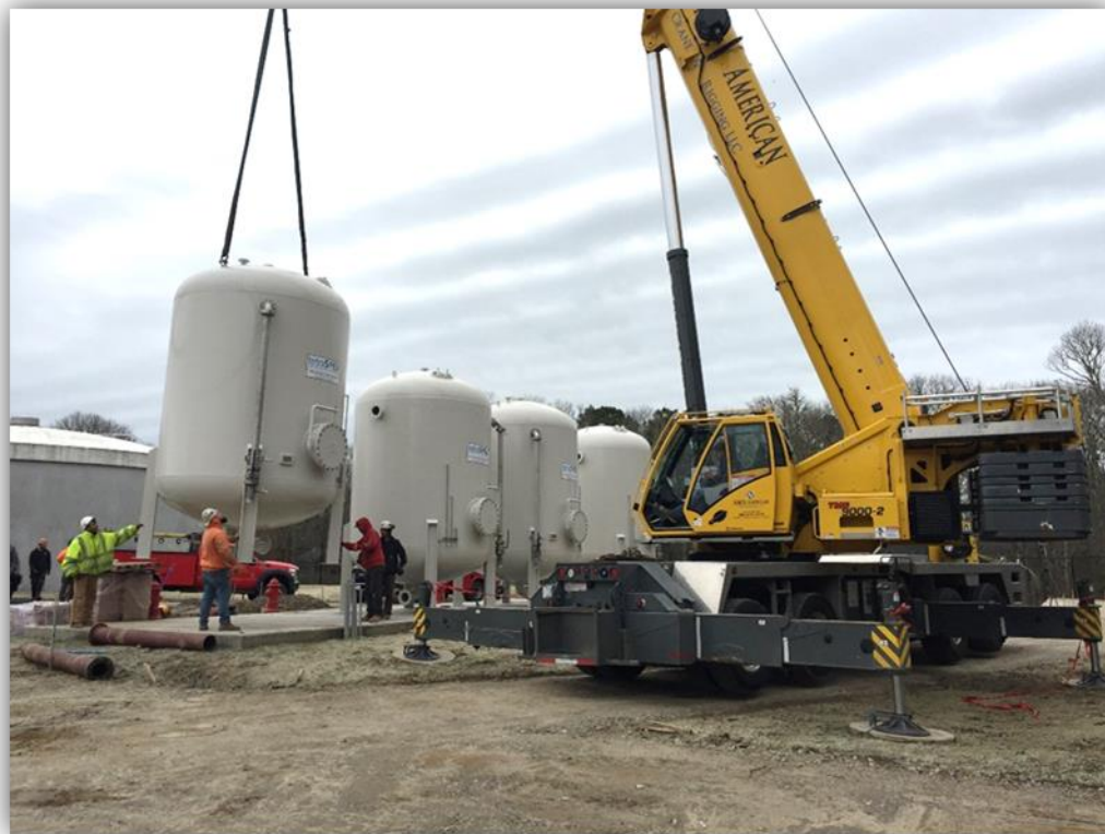
GAC contactors being installed in Barnstable
