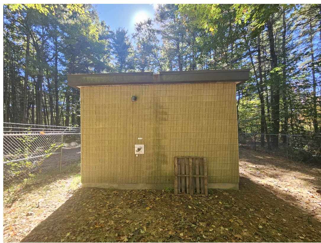
6. NORTHEAST CORNER OF BUILDING FACING SOUTHWEST
