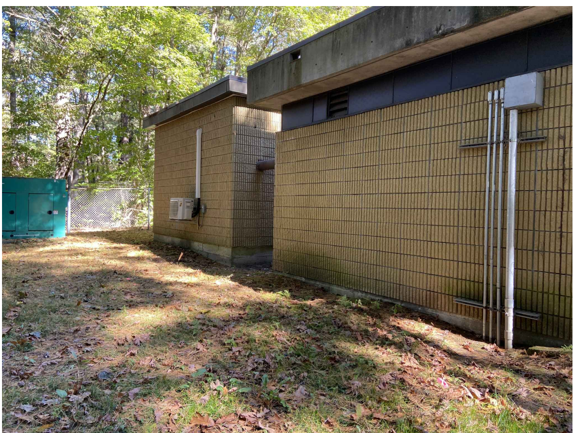
8. NORTHEAST CORNER OF FACILITY OUTSIDE OF FENCE FACING SOUTHWEST
