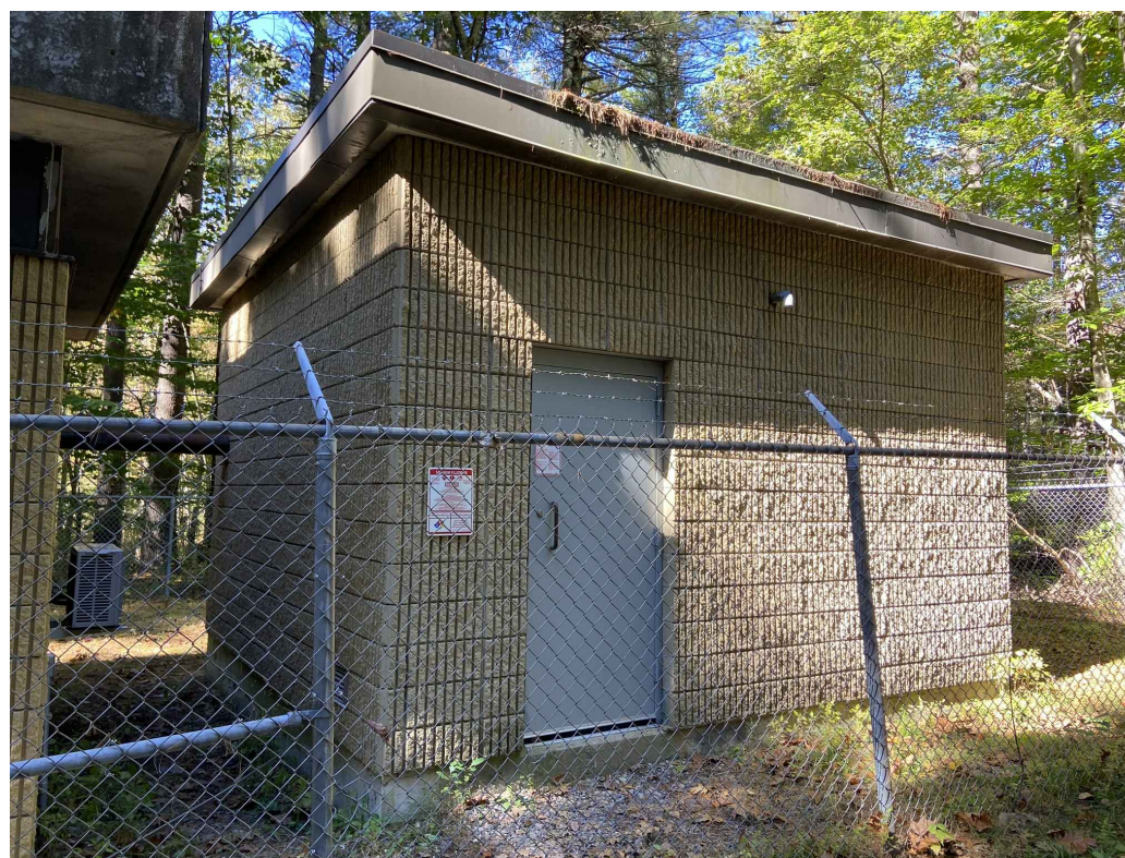
3. SOUTHWEST CORNER OF BUILDING FACING NORTHEAST
