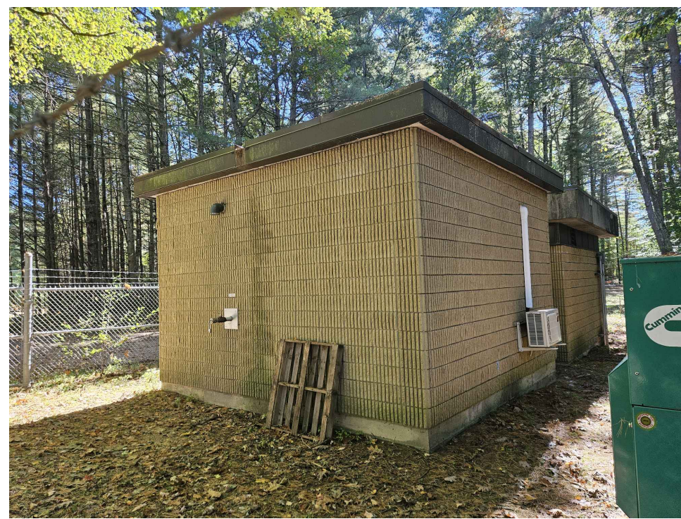
2. NORTH SIDE OF BUILDING FACING SOUTHEAST
