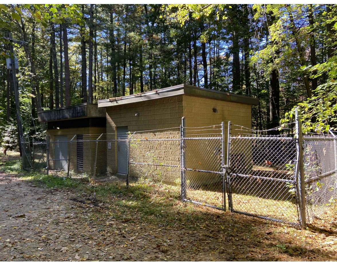
4. NORTHEAST CORNER OF FACILITY OUTSIDE OF FENCE FACING SOUTHWEST
