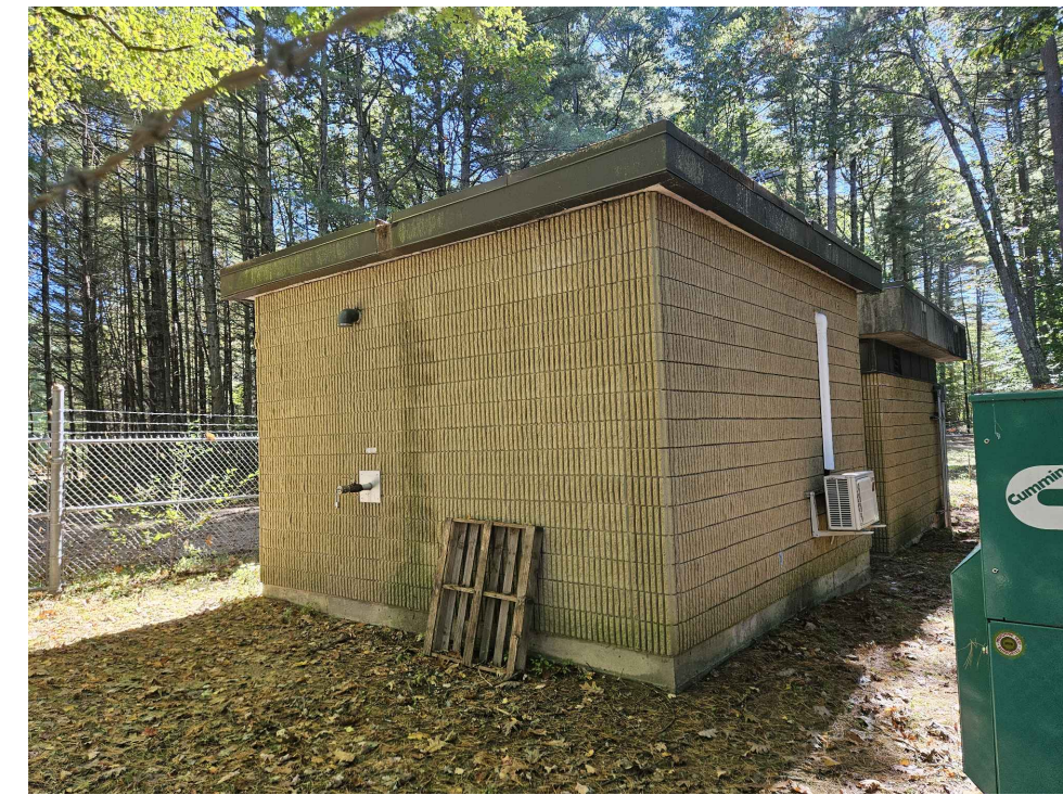
2. NORTH SIDE OF BUILDING FACING SOUTHEAST
