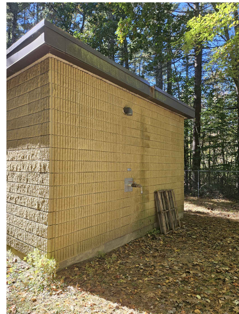
6. NORTHEAST CORNER OF BUILDING FACING SOUTHWEST
