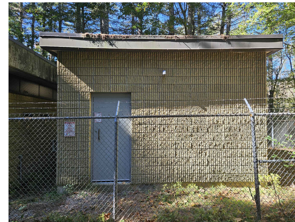
5. EAST SIDE OF BUILDING FACING WEST
