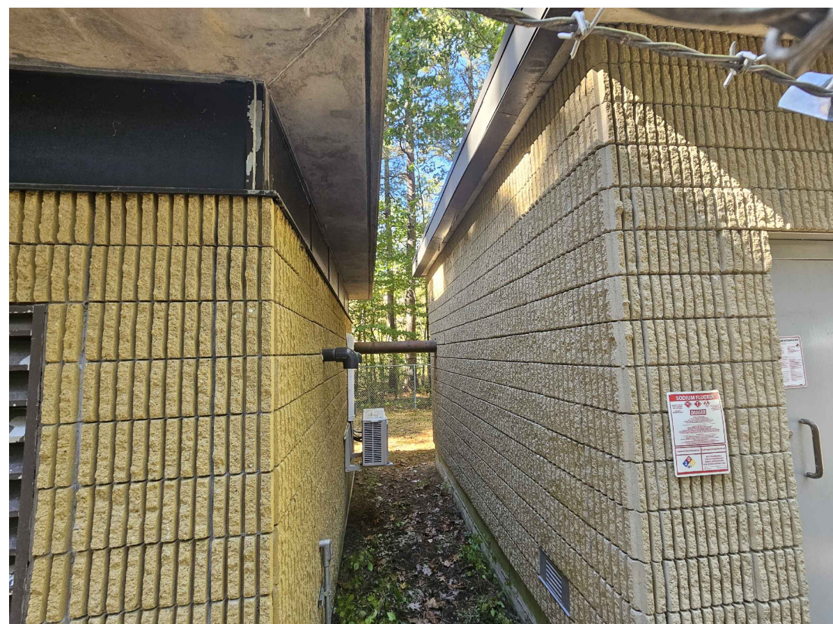
7. EAST SIDE OF PIPING BETWEEN CHEMICAL FEED BUILDING AND WELL PUMP HOUSE FACING WEST
