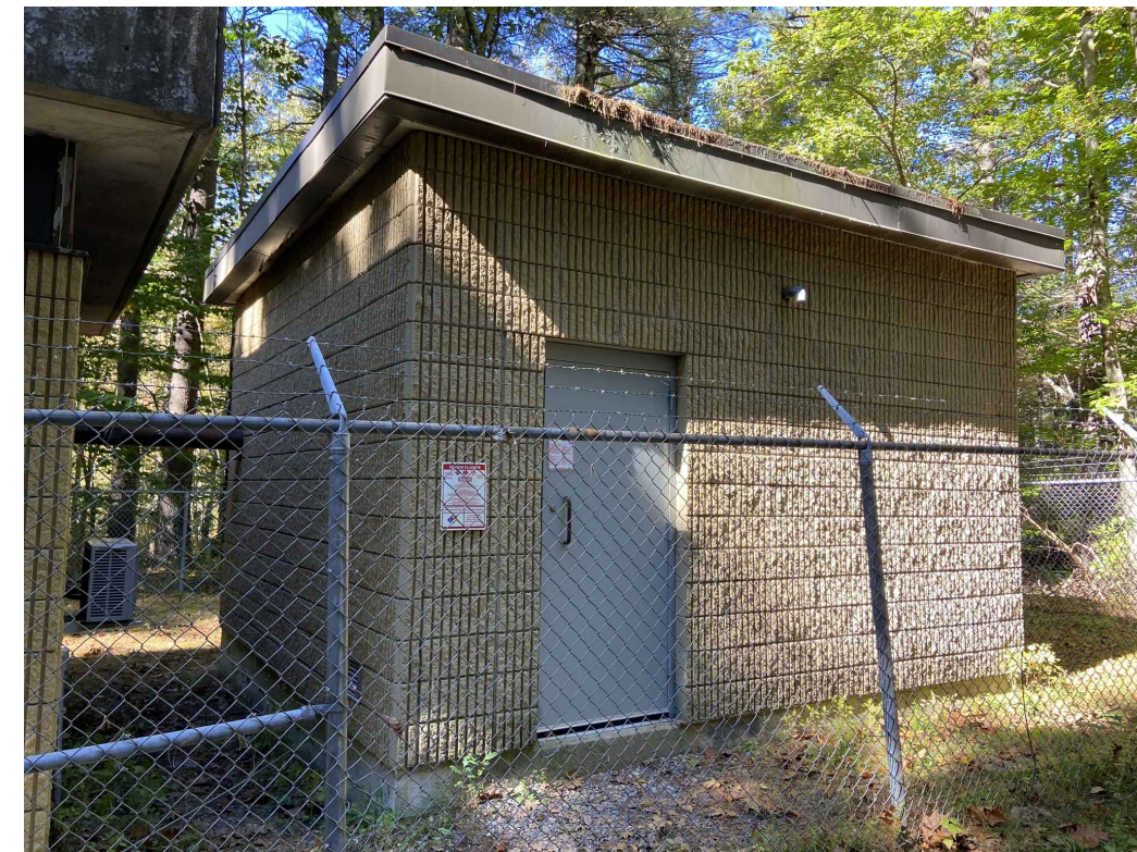
4. SOUTHEAST CORNER OF BUILDING FACING NORTHWEST
