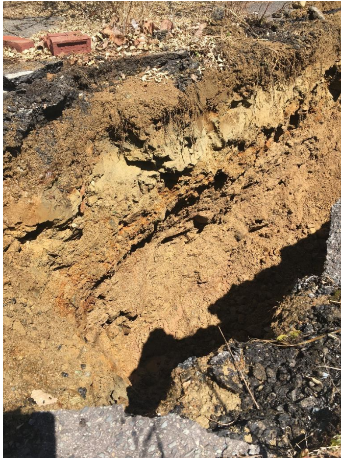
Second test pit in Infil-200, note 20" of fill mottles at 36"
