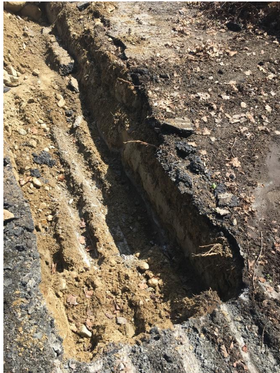
Concrete slab encountered 12" below surface near Basin 1
