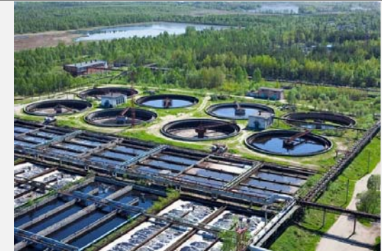
Wastewater Treatment Odors
