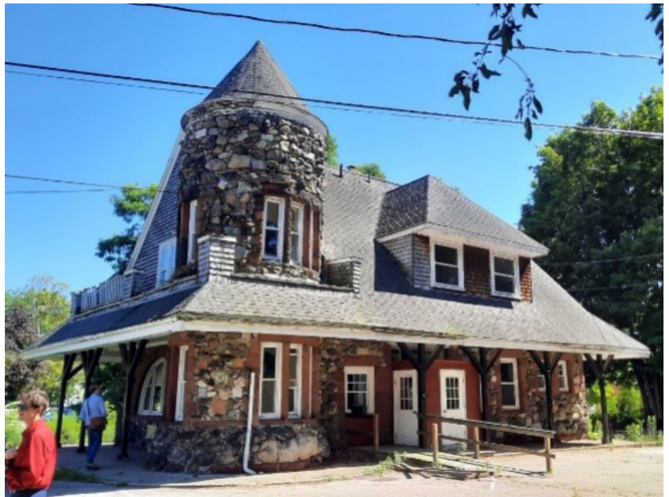
Panelists touring the Lansing Millis Memorial Building/Train Depot. Source: TAP Panel.
