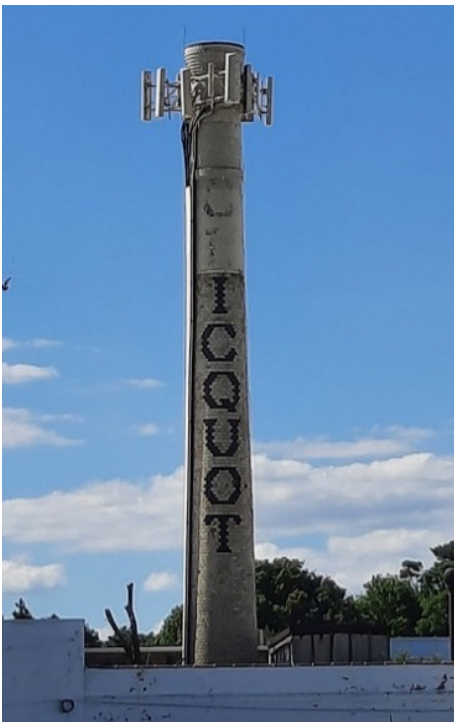
Clicquot Chimney. Source: TAP Panel.
