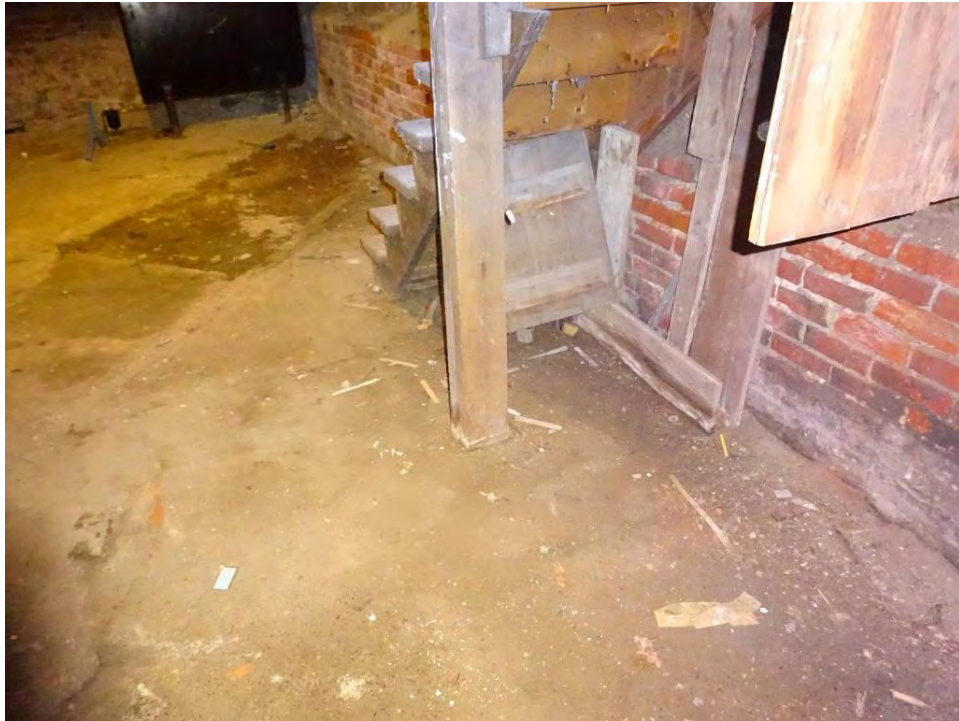
Photo 5 Wood post at corner of basement stair
