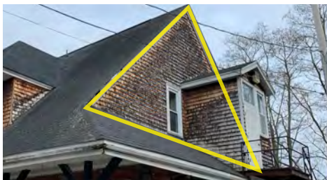
The east and west gable ends match the pitch of the hip roof
