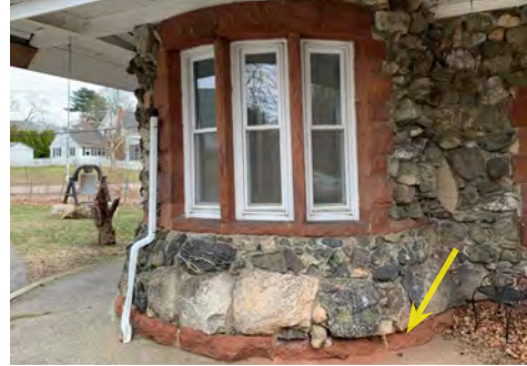
Red sandstone foundations are spalling throughout
