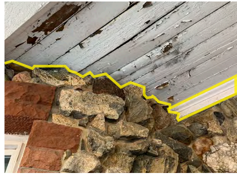
Soffits are carefully cut at turret, with moldings elsewhere
