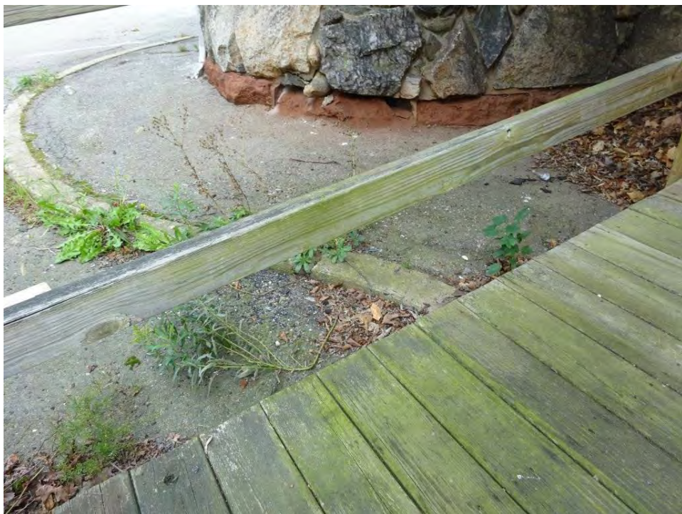
Photo 12 Deteriorated brownstone sills at base of walls at north elevation
