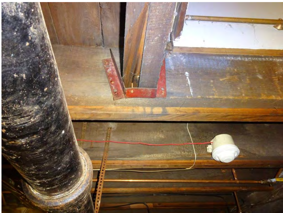
Photo 6 Improperly installed hanger at stair header-trimmer connection
