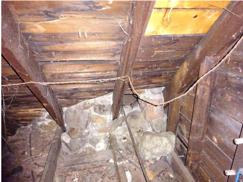
Photo 9 Dislodged stone at south edge of turret at roof level
