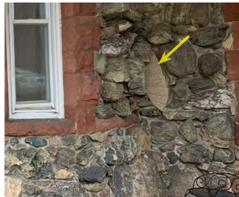
An inscribed millstone embedded in the masonry at the turret
