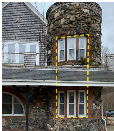
Masonry openings at turret are vertically-aligned
