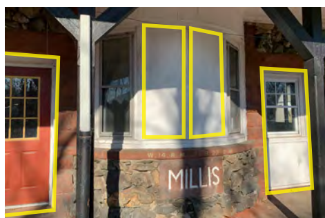
Bay window at south wall, abutted by twin masonry openings
