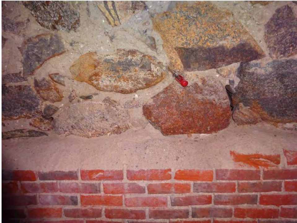
Photo 7 Interior face of stone foundation wall
