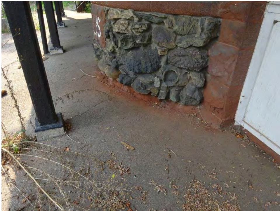
Photo 11 Deteriorated brownstone sills at base of walls at south elevation
