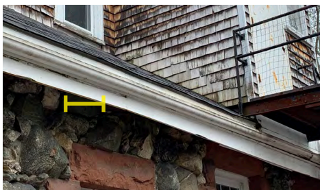
Smaller overhang at west end, compared to other three sides
